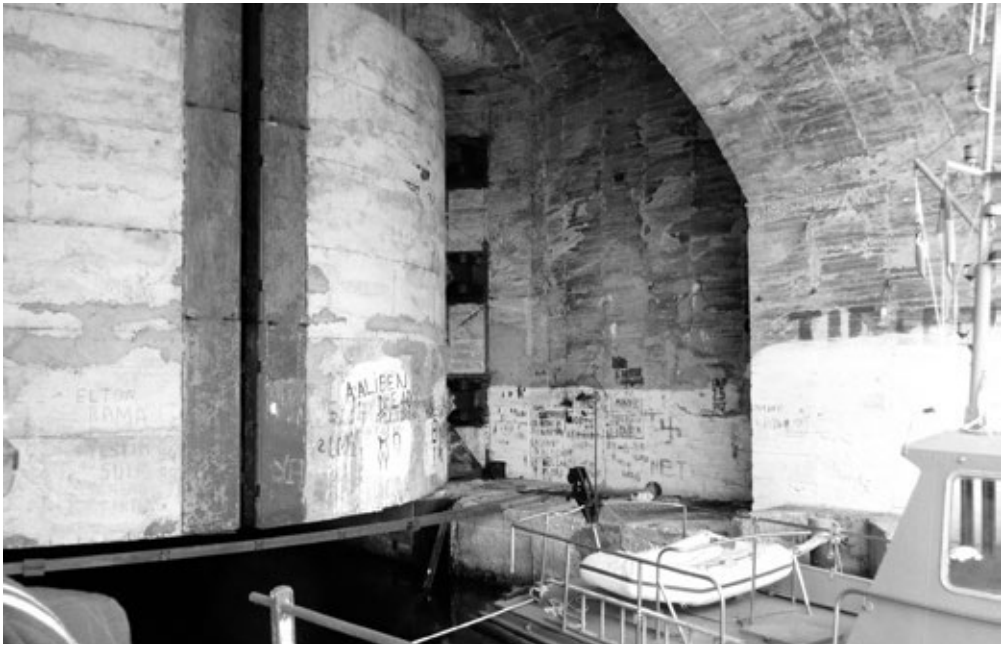
Reinforced main entrance door of Panorma Tunnel, 2010 (Ph. Studio Terragni Architetti)
